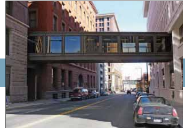
Figure 3.13 The existing condition along 4th Street.
