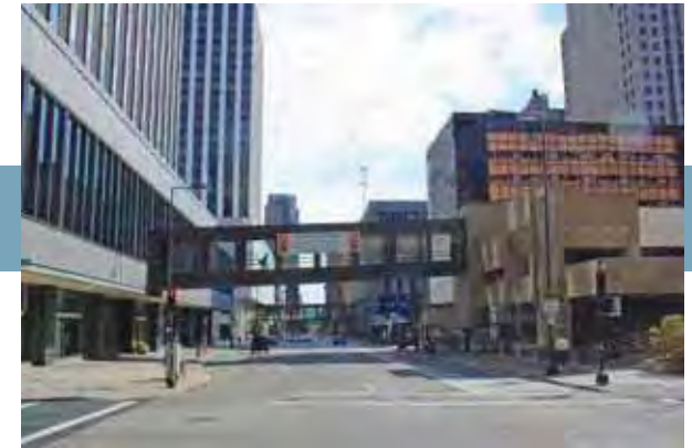
Figure 3.1 The existing condition of the northern edge of the Central Station block.
