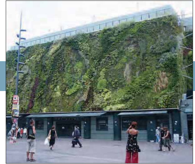
Figure 3.9 The creation of a green “living” wall on the OMF along Prince Street would help to soften the edge of the facility.
