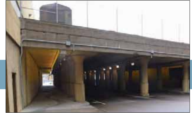
Figure 3.15 The existing condition of the Sibley viaduct.
