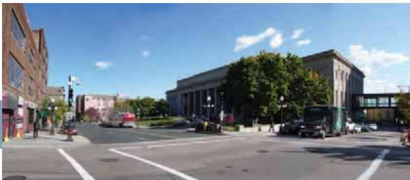
Figure 3.5 The existing condition of Union Depot.
